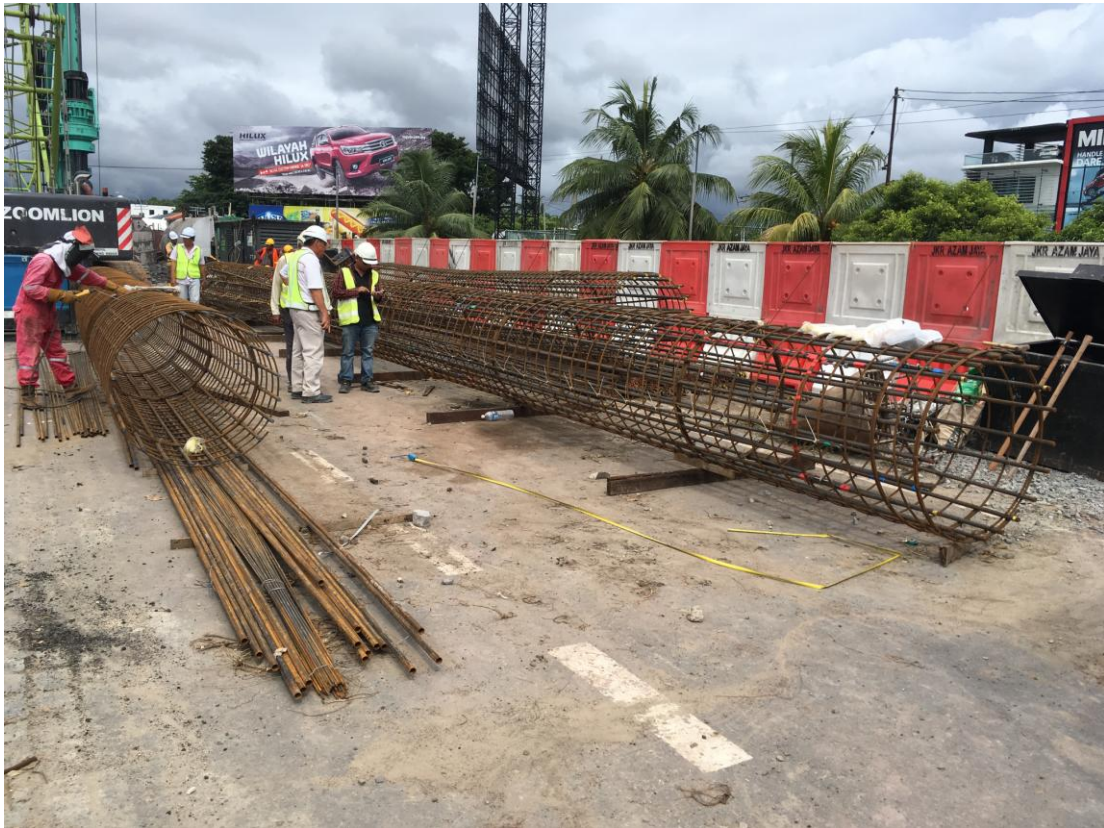
Photo 7: Inspection of Steel Cages
