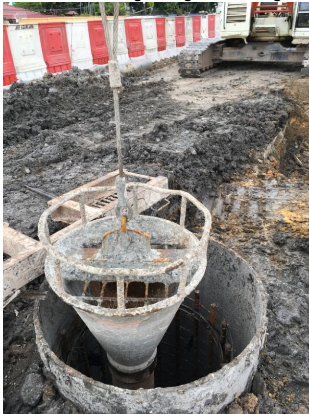
Photo 10: Full length Steel Cages and Tremie Pipe were installed for PDA pile
