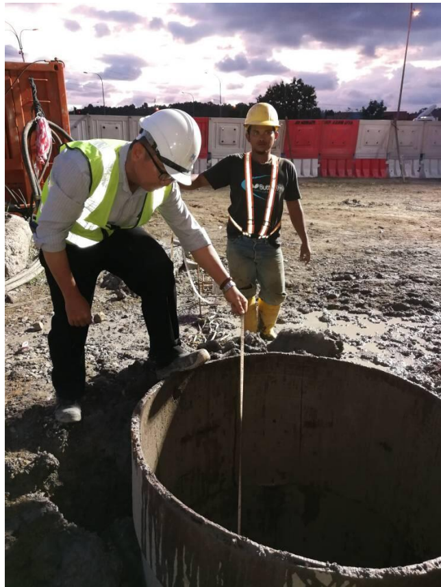
Photo 6: Confirmed Pile Toe Level after Cleaning Base
