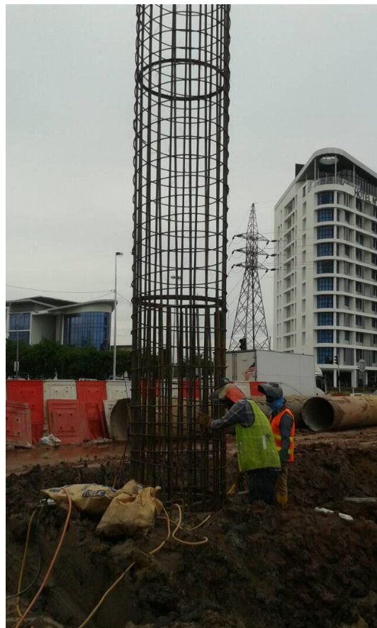
Photo 8: Jointing of steel cages , 2m lapping length of starter bars by welding
