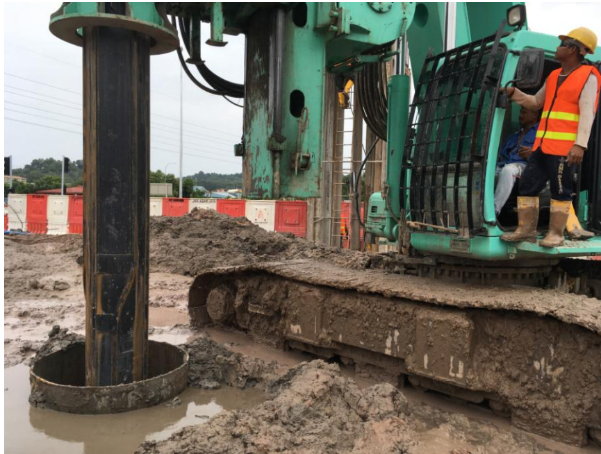
Photo 3: J5- Boring Works
