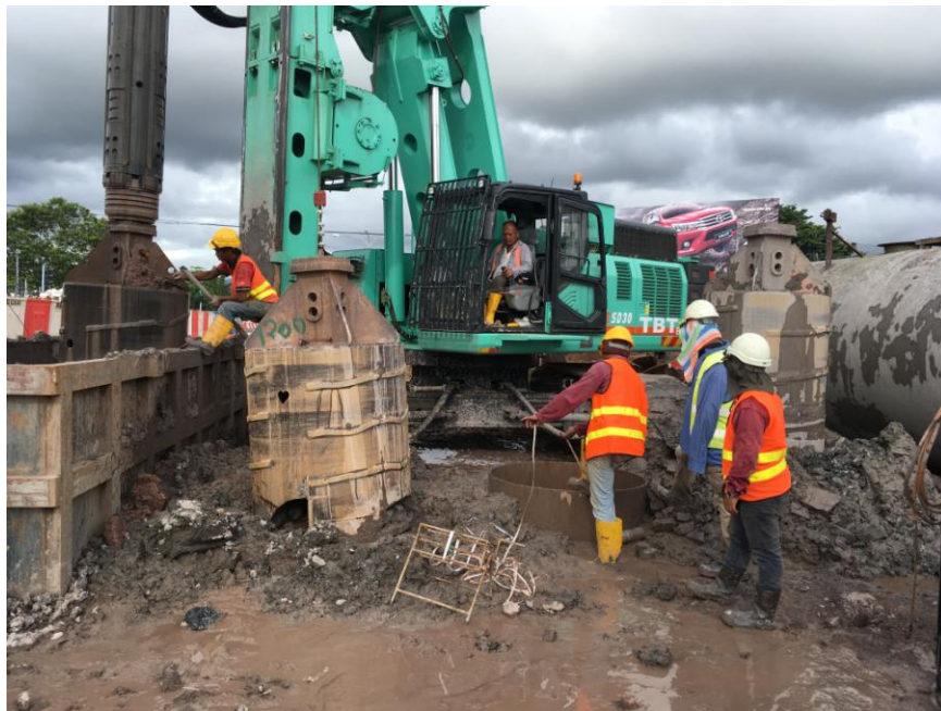
Photo 4: J6- Boring Works
