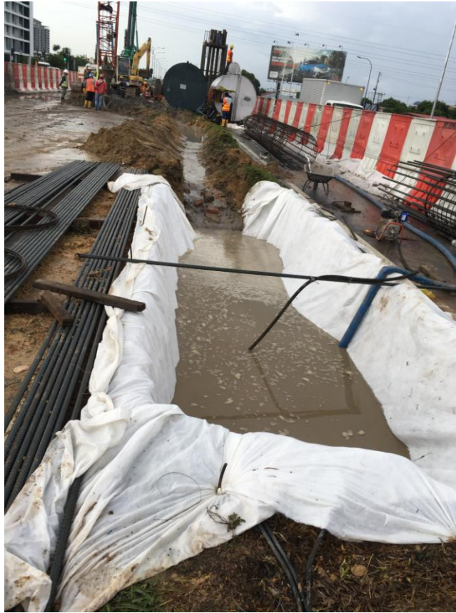
Photo 13: Temporary Storage Pond (filter cloth) for water before pumping to storage tank
