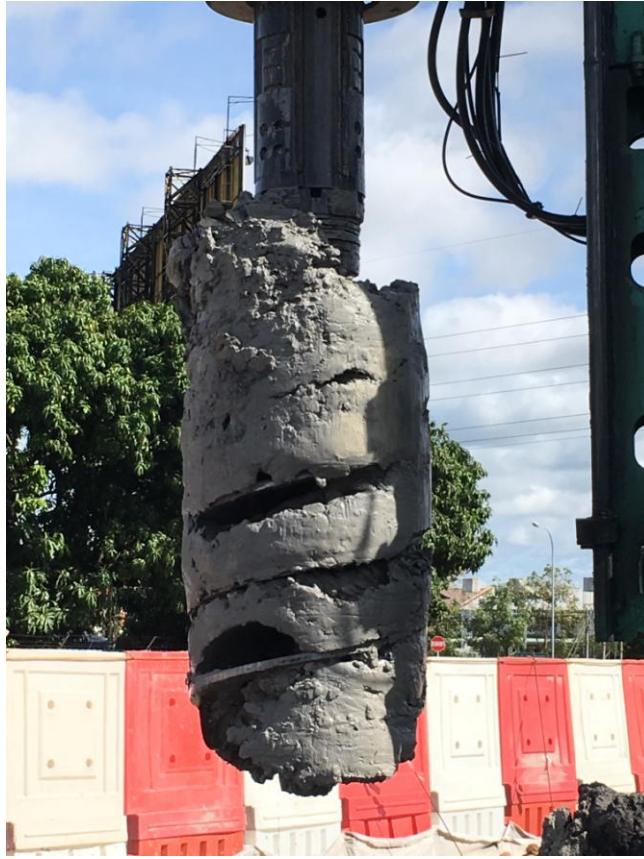
Photo 5: Bored out soil/rock using Rock Auger
