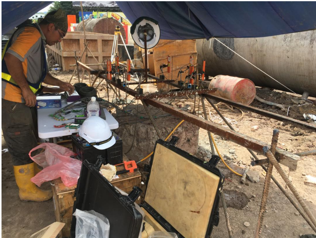
Photo 16: J6- Instrumented Bi-Directional Load Test (BDLT)
