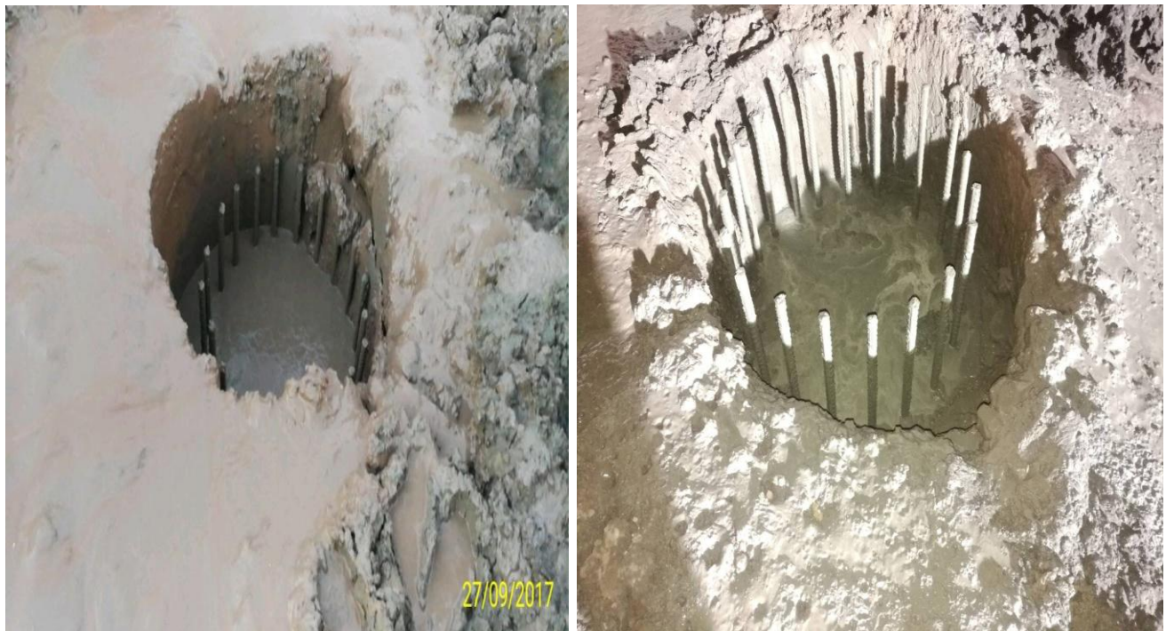
Photo 12: Borehole after Temporary Casing was Extracted
