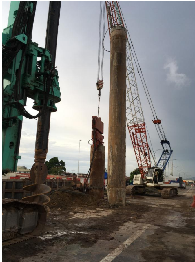
Photo 2: Installation Temporary Casing by 7 tons Double Jaws Vibro Hammer
