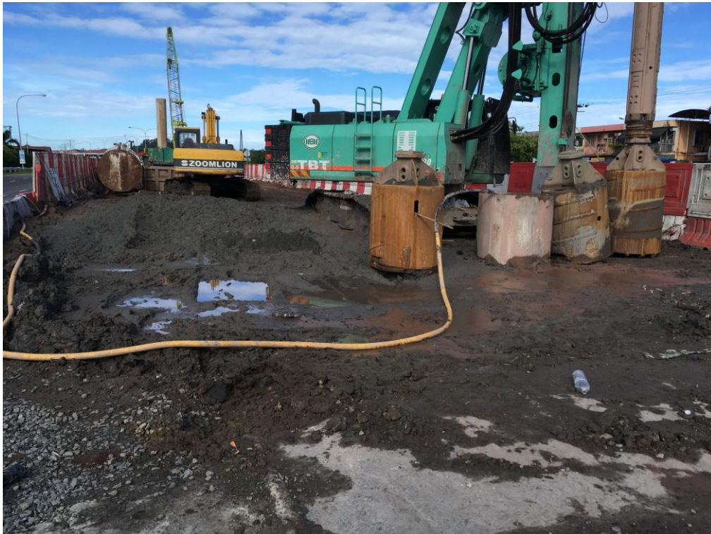
Photo 14: Boring tools (Boring & Coring Bucket and Cleaning Bucket), Water from storage tank supplying to borehole
