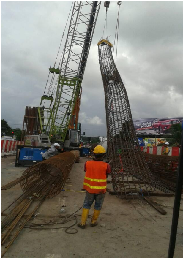
Photo 9: Hoisting/lifting of Steel Cages
